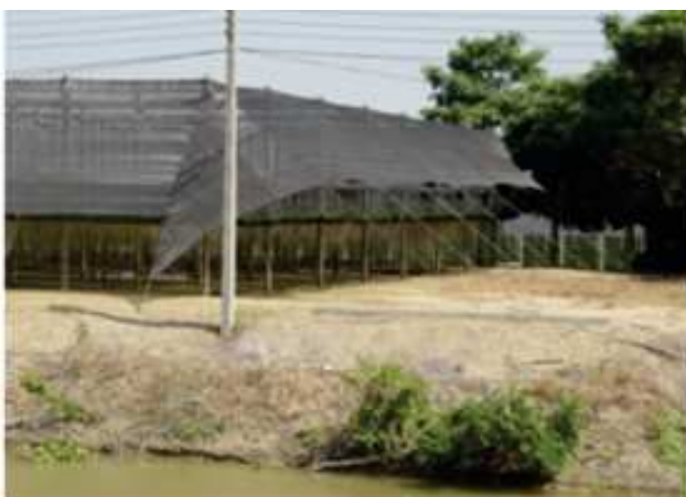
Fig. 4. A greenhouse is open at the sides to facilitate proper air circulation and to prevent heat accumulation.
